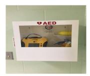
An automated external defibrillator (AED) is a lightweight, portable device that delivers an electric shock through the chest to the heart. The shock can stop an irregular heart rhythm and allow a normal rhythm to resume following sudden cardiac arrest. Sudden cardiac arrest is an abrupt loss of heart function. If it's not treated within minutes, it quickly leads to death. With simple audio and visual commands, AEDs are designed to be simple for use.
